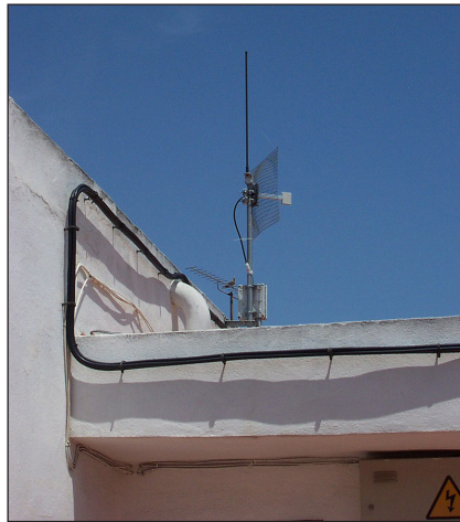
Parabolic dishes transmit and receive the radio waves only in particular directions and can give much greater range than omnidirection antennas.
