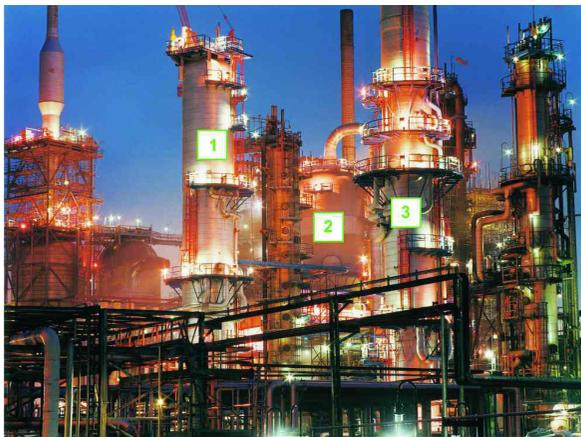
Part of the catalytic cracker at Fawley in the south of England. 1 Fractionating column to remove and recover the butanes. 2 The catalyst regenerator. 3 Fractionating column to remove and recover ethane.
