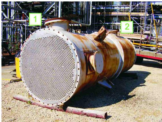
This exchanger is used for cooling product with water which enters the shell side at 1 and leaves at 2. The product to be cooled flows through the small tubes. The exchanger has been taken out of service to clean the tubes to improve the efficiency of the cooling process.
