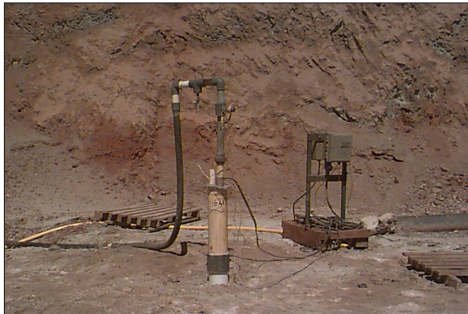
Recovery well at former San Manuel operation.
