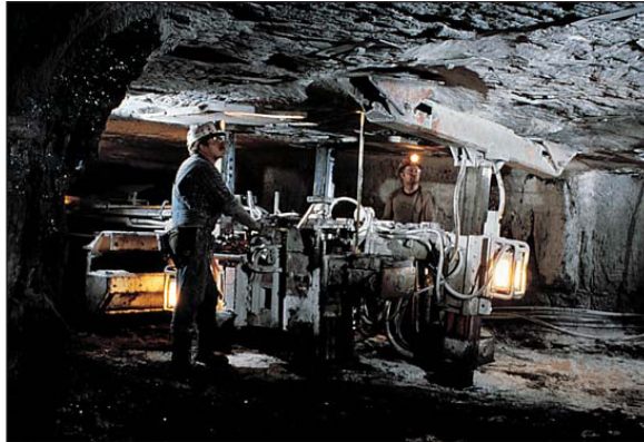
Inserting steel bolts to support the roof of an underground.
