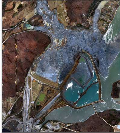
Aerial photograph of Kingston Fossil Plant coal fly ash slurry spill site taken the day after the event.
