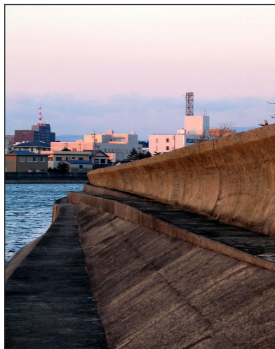
Tsunami wall at Tsu, Japan.
