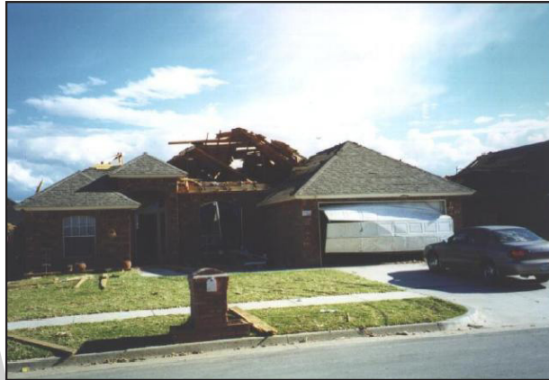
A house displaying EF1 damage. The roof and garage door have been damaged, but walls and supporting structures are still intact.
