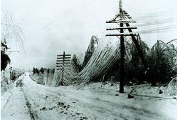
Power lines sagging after an ice storm. Besides disrupting transportation, ice storms can disrupt utilities by snapping lines and poles.
