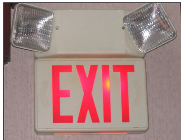
An exit sign in the United States, showing the way to the nearest exit, with two emergency lights for electrical failure.
