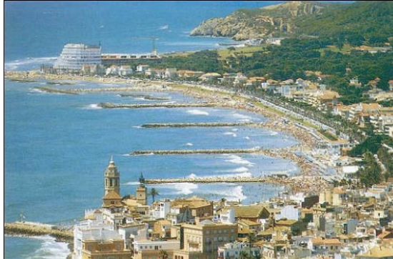
Groynes are engineered structures that aim to prevent erosion of the beach front.
