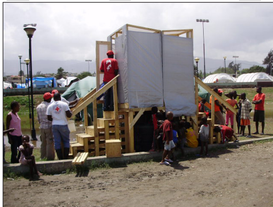
Emergency toilet in Haiti, suitable for areas where digging pit latrines is not possible.
