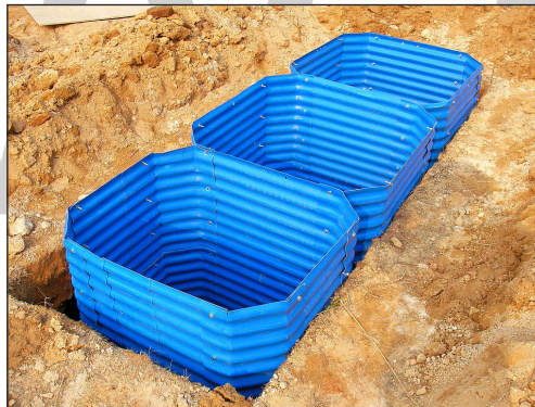
Emergency pit lining kits, suitable for areas with high water table.
