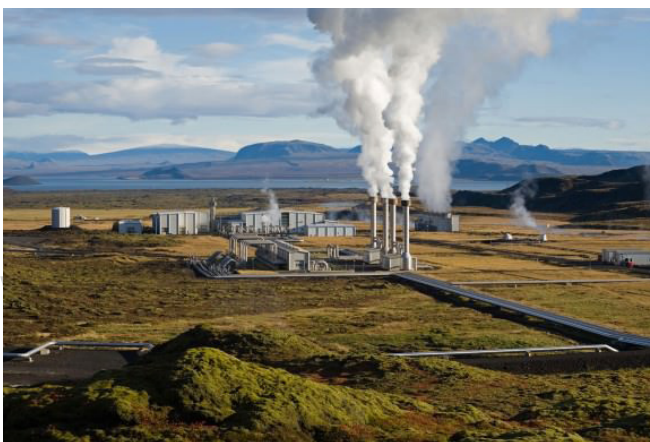
Steam rising from the Nesjavellir Geothermal Power Station in Iceland.
