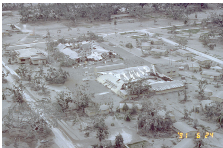
Buildings and vegetation at Clark Air Base, Philippines, destroyed by a thick, wet layer of ash following the gigantic explosion of Mount Pinatubo.
