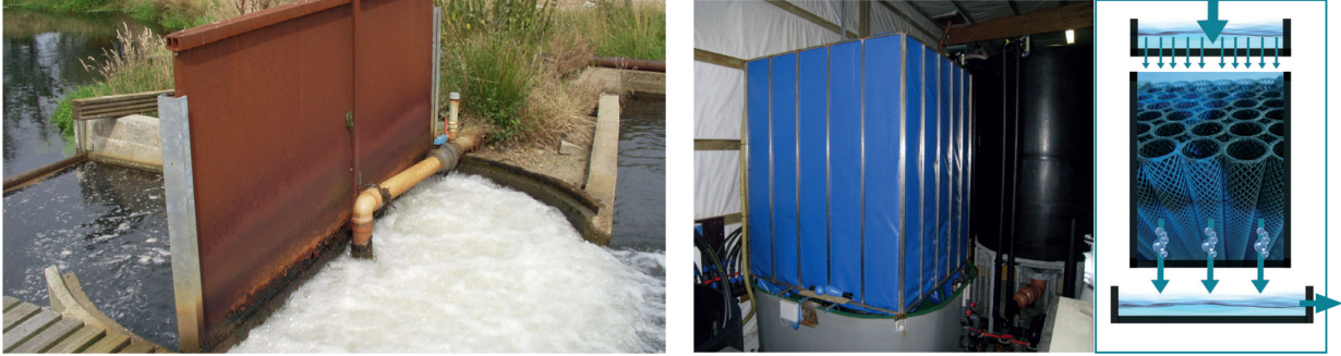
Figure: Trickling filter wrapped in a blue plastic liner to eliminate splashing on the floor. The aeration/stripping process is also called \text{CO}_2 -stripping. The media in the trickling filter typically consists of the same type of media as used in fixed bed biofilters
