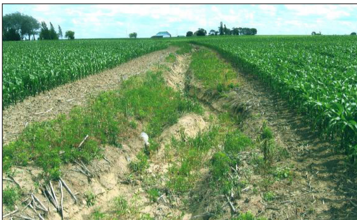
Gully erosion may develop in locations where rill erosion has not been managed.
