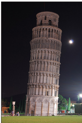
The Leaning Tower of Pisa— an example of a problem due to deformation of soil.
