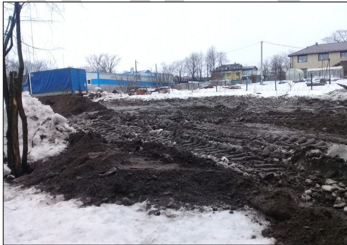
Exposure of soil at a construction site creates potential for soil erosion by water, wind, or both. Eroded soil pollutes waterways and causes sedimentation of ponds and reservoirs.
