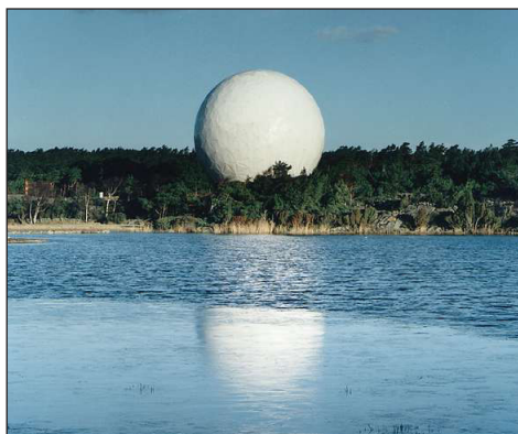
The 20-metre (60-foot) diameter, radome-enclosed, millimetre-wave telescope.
