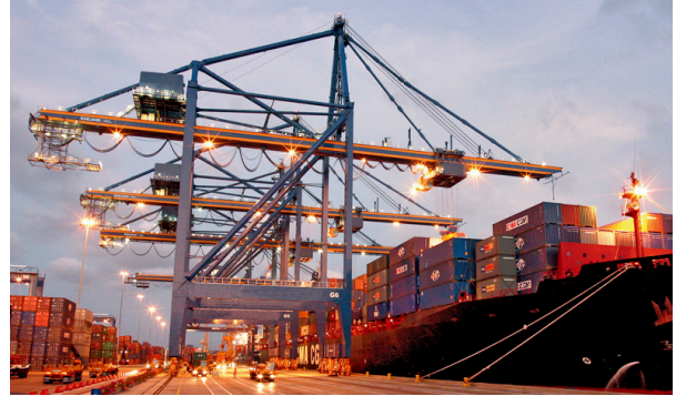
AGV and gantry crane used for loading containers on ships
