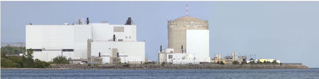
The Darlington nuclear power plant in Ontario produces power from four 878 MW CANDU reactors.
