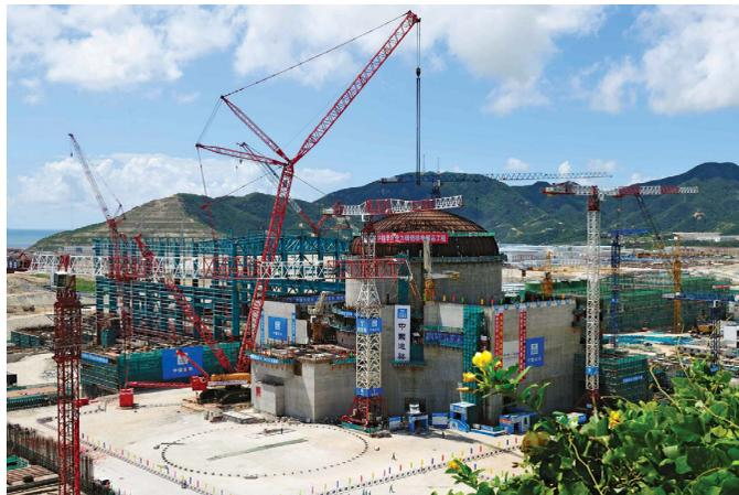
Installation of the dome of a containment structure at the Taishan nuclear power plant.
