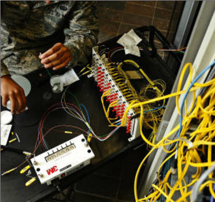
Working on fiber-optic cables.
