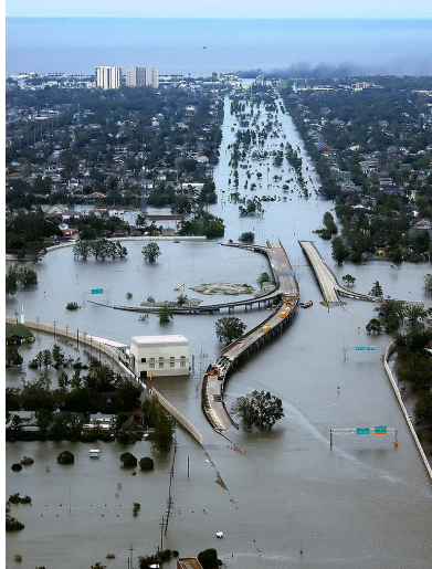
Significant flooding in New Orleans as a result of Hurricane Katrina and the failure of the city's flood protection systems.
