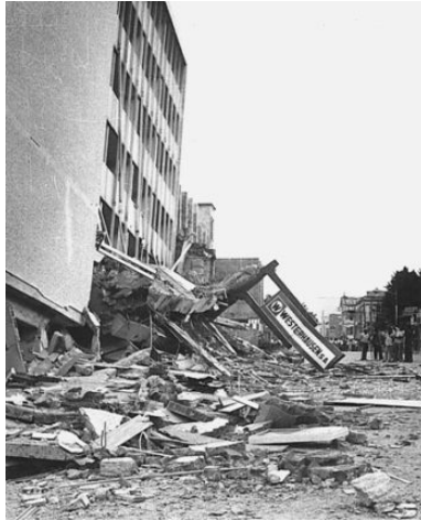
Collapsed Gran Hotel building in the San Salvador metropolis, after the shallow 1986 San Salvador earthquake.
