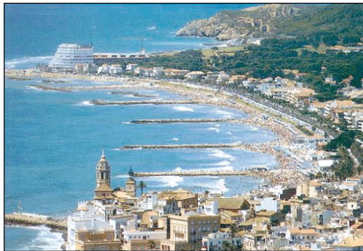
Groynes are engineered structures that aim to prevent erosion of the beach front.
