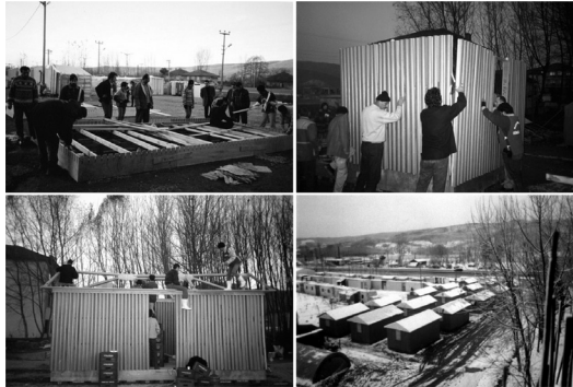
Kit solutions: assembly process by local community and cluster of the Paper Log Houses designed by Shigeru Ban.
