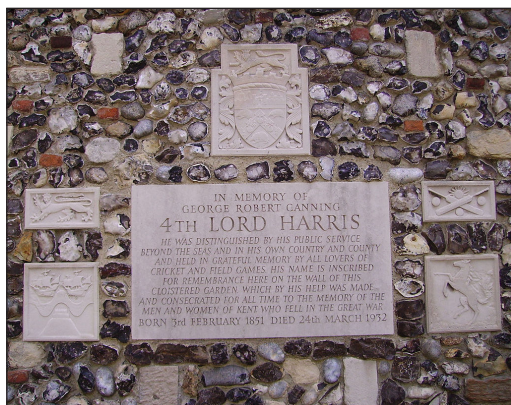
A typical medieval wall (with modern memorial) at Canterbury Cathedral – knapped and unknapped (“cobble”) flints are mixed with pieces of brick and other stones.
