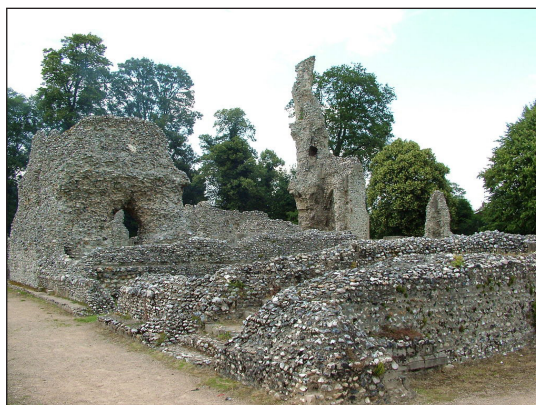
Ruins of Thetford Priory show flints and mortar through the whole depth of the wall.
