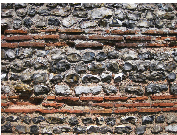
Close-up of the wall of the Roman shore fort at Burgh Castle, Norfolk, showing alternating courses of flint and brick.
