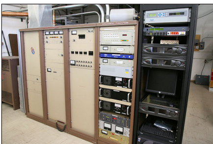
35 kW, Continental 816R-5B FM transmitter, belonging to American FM radio station KWNR broadcasting on 95.5 MHz in Las Vegas.
