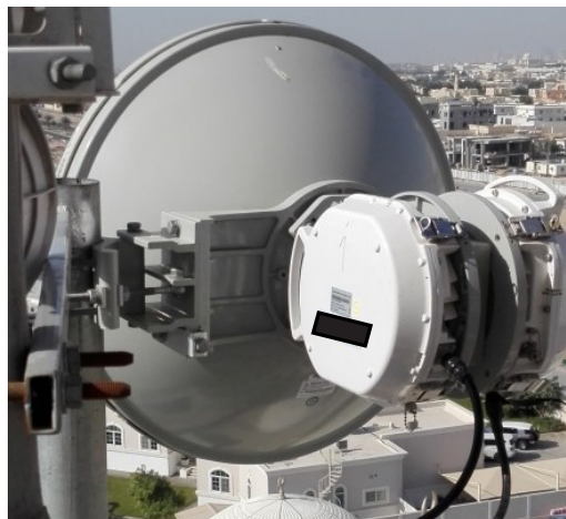
CableFree 2+0 XPIC Microwave Link showing OMT and two ODUs connected to H & V polarity ports.
