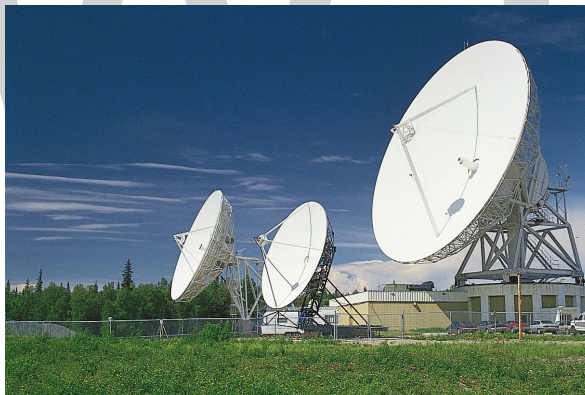
Radio wave dish-type antennas, varying in diameter from 8 to 30 metres (26 to 98 feet), serving an Earth station in a satellite communications network.
