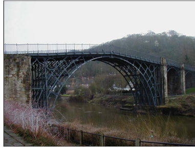
Ironbridge, made of cast iron.
