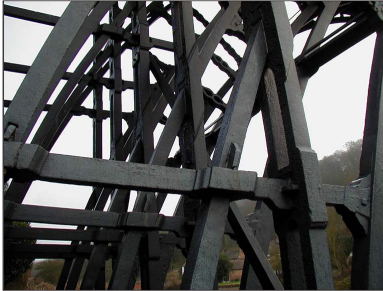
Ironbridge, made of cast iron.
