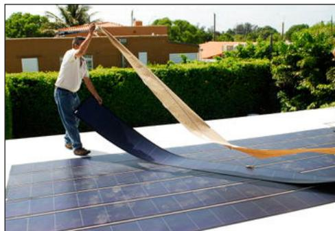
A thin film solar panel composed of non-crystalline silicon deposited on a flexible material.
