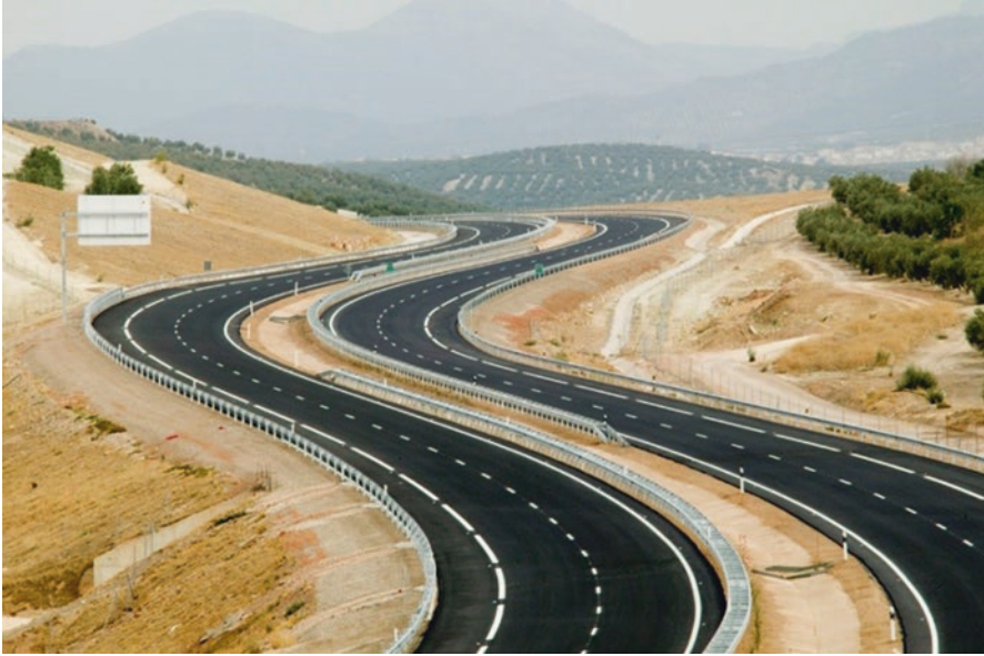
Fig. 11.1 Infrastructural white elephants in Spain: extensive motorway network. Source: By Gestion.Inf.And. – Own work. Used under Creative Commons Attribution 3.0 Unported. Retrieved from https://commons.wikimedia.org/w/index.php?curid=6026287
