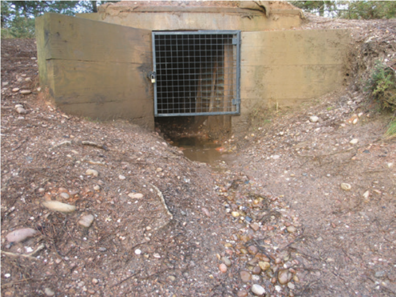
Figure 3.9A Exit of dry tunnel
