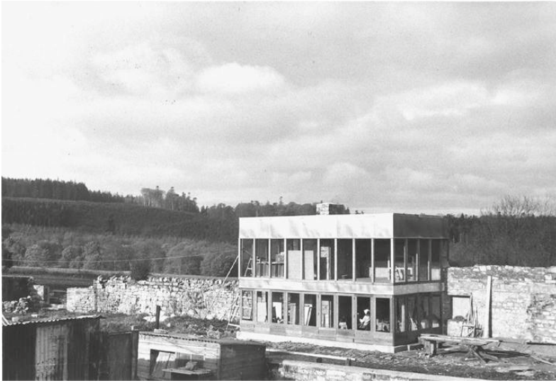
Fig. 19.4 Upper Lawn under construction looking north-west.
